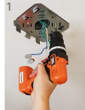
1 Mount plate to junction box.
