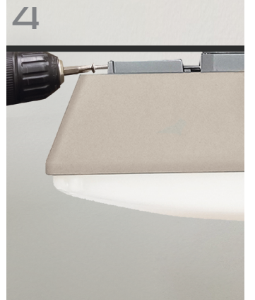
4 Two mounting screws close and secure fixture to the mounting bracket.
