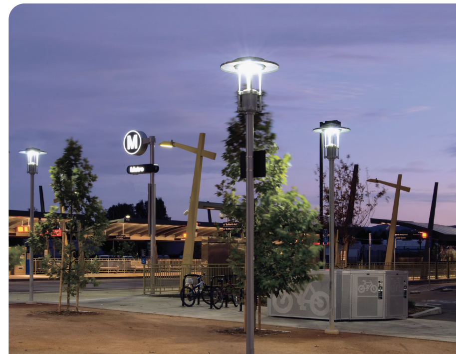
For a seamless look from parking lot to entry way, look to the Era and Bounce families for a comprehensive site lighting solution.
