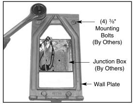
2. Securely mount wall plate over junction box (by others) on wall. **Note: Hardware provided by others.**
