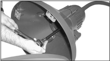
2. Install fixture head to crook arm with lock washers & nuts, tighten to 20 ft-lbs. Make sure fixture aligns with crook arm. **NOTE:** Orient "hinge" side of fixture towards pole.
