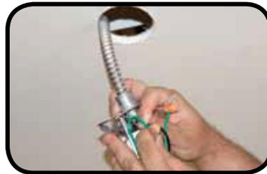
Pull the pre-existing wiring below the ceiling and connect to the J-tube assembly through the 1/2" knockout. A 3/8" flex conduit duplex connector may be used to easily daisy chain fixtures together. For end-of-run applications, a standard 1/2" connector can be used.
