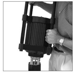
**4.** Install fixture assembly to pole. Orient fixture relative to mount to provide desired lighting distribution.
