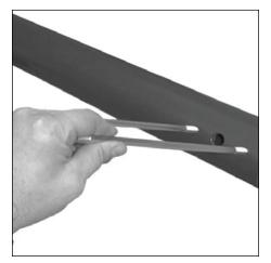
Place backing plate inside pole and thread long threaded end of studs into backing plate.
