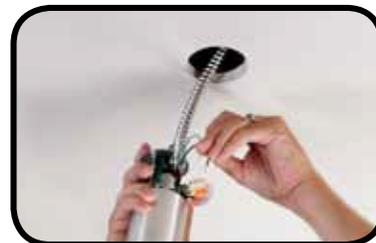
5. Feed the wired J-tube assembly through the ceiling cutout. The J-tube assembly has been designed to conveniently lie on top of the ceiling material. (NOTE: This fixture is designed for use in a non-insulated ceiling.)
