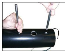
4. Insert pole-backing plate through top of pole. Align three holes in pole with matching holes in backing plate. Insert both draw bolts into pole holes and thread draw bolts into the backing plate.
