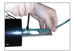
**3.** Lay pole horizontal on padded supports to protect finish. Pull field wires through pole and out the top. Tie-wrap wires to pole backing plate. Tie field wires in a knot or back loop through tie-wrap. Wire leads need to extend 12" beyond the pole top.
