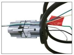
**2.** Feed pole wire leads going inside the spreader retainer springs and up through the holes into the wire chamber and out the chamber mouth. Connect field wire leads to fixture leads observing polarity, i.e., ground-to-green, white-to-common, and black-to-voltage.
