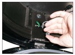
7. Fit one washer and jam nut onto each draw bolt, but do not tighten, Square the fixture carefully to the pole; tighten jam nuts. Attach securing nuts with a minimum of 15-20 ft lbs torque to all nuts. If fixture is not level after pole is erected, loosen all four nuts. Re-tighten nuts after final leveling using the above procedure.
