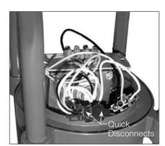
**12.** Connect quick-disconnects (2), and tuck into driver compartment. Connect fixture leads to field circuit wires at handhole observing polarity, i.e.; green-to-ground, white-to-common, and black-to-voltage.
