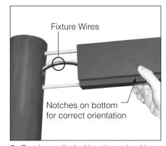
**3.** Feed supplied wiring through wiring hole in pole and through handhole. Slide arm onto studs with the notches downward.
