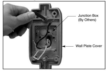
1. Securely mount wall plate over junction box on wall. **CAUTION: Structural integrity of mounting plate** attachment to wall is by others.
