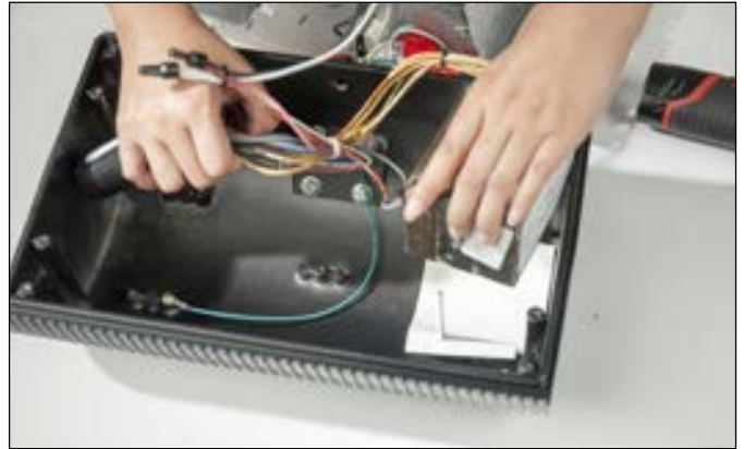
12. Remove ballast assembly from housing, (Note: There will be 2 wires, black and white from the housing arm, that will prevent the assembly from being removed. Cut these two wires from the ballast assembly, but keep about 6" of this wire coming from the arm opening. Properly discard ballast assembly.
