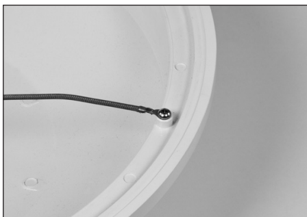
10. Use ring terminal and ground to fixture housing and top cover.
