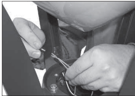
23. Pull green ground wire from arm until it's within fixture hub and connect to green ground wire installed on step 6 above with the supplied wire nut.
