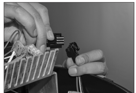
9. Connect TIR Light engine quick disconnect to fixture quick disconnect. If the input connectors on the kit assembly do not match the connector in the field, please use UL listed connectors to make the connection.
