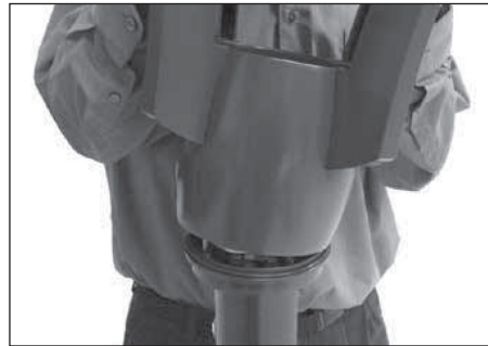
20. Install fixture onto base, orient fixture relative to mount in order to provide desired lighting distribution.
