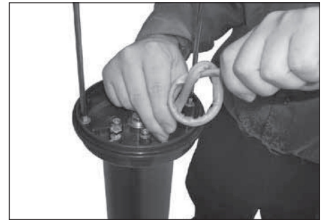
18. Tie pole wiring into a knot in order to prevent it from dropping through the wire-way hole.
