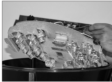
2. Disconnect the HID Reflector/Emitter deck and remove HID Reflector/Emitter deck assembly.
