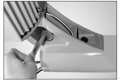
2. Attach fixture assembly to pole (2 places) using washer and C" bolt. Be sure fixture is aligned with anchor base and other fixtures for multiple mounts. Tighten to 20 ft.-lbs. using N" socket wrench.
