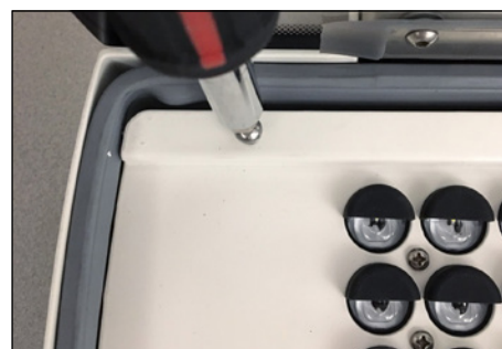
9. Install (4) screws from bezel assembly to housing. Self threading TORX screws are provided if existing fixture housing bosses are not threaded.
