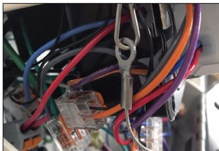
5. Attach driver assembly retention cable.
