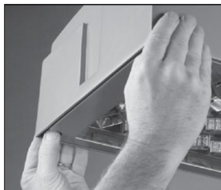
2. On the fixture, push up on door frame and push both spring tabs simultaneously outward using thumbs.
