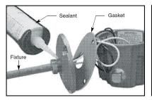
1. Install fixture, coating exposed threads with sealant to keep moisture from entering junction box.
