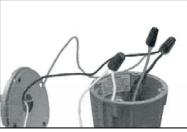
2. Connect fixture leads to circuit leads observing polarity, i.e.; braided bare copper-to-ground, white-to-common and black-to-voltage.
