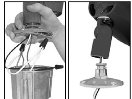
3. Install fixture onto coupling. Attach fixture leads observing polarity, i.e.; green-to-ground, white-to-common, and black-to-voltage.
