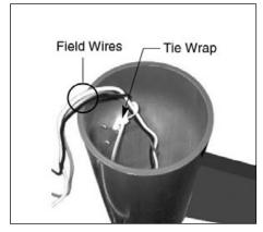
**4.** Pull field wires through pole tenon into slipfitter and through tie wrap. Tie field wires into a knot or back loop through tie wrap.
