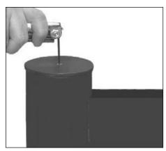
**7.** Make connection to field wires at top of slipfitter. Replace pole cap.
