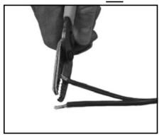
1. Cut main cable at desired branch location. Slit cable ends approx. 2". Strip all cable ends 3/8".
