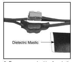
3. Remove paper backing from both sides of dielectric mastic. Stretch one piece of dielectric mastic around each wire connector, molding it around connectors and cables so they are completely watertight.
