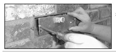
Attach fixture wires to field wires using U.L. approved wire nuts ensuring correct polarity, i.e., green-to-ground white-to-common, black-to-voltage. Install ballast / socket plate and tighten screws securely. Install lamp of type and wattage as shown on fixture label and chart on this page (not needed for L.E.D. fixture).
