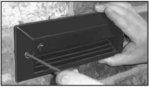
Install face plate/gasket assembly and secure with screws.
