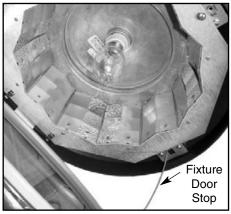
5. Install lamp of type and wattage shown on fixture label.
