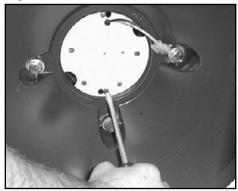
Install fixture head to arm with washers & nuts, tighten to 20 ft.-lbs.
