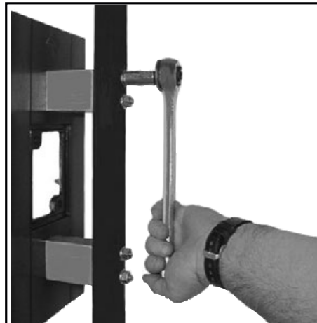
11. Install crook arm onto bolts and secure with washers and nuts. Tighten to 20 ft.-lbs.
