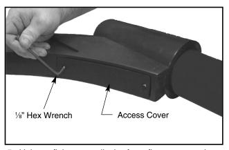
Using a fish tape pull wire from fitter top to pole handhole. Install access cover and secure with screws.
