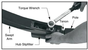
3. Install swept arm to hub with (2) bolts, tighten to 20 ft.-lbs.
