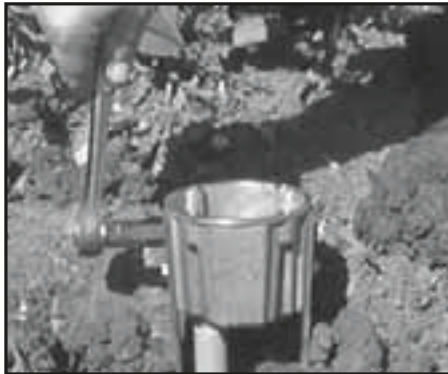
2. Connect junction box to conduit system. Attach stakes (2) to side of junction box with screws provided. Thread sealant must be used to prevent water entry.
