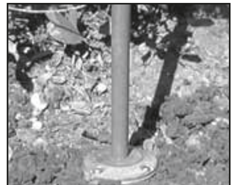
6. Junction box cover must be slightly above grade level.
