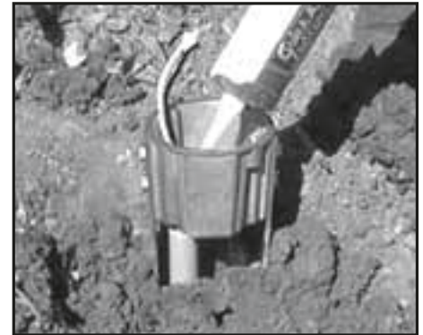
3. Bring wires through and seal conduit entries inside junction box with good grade RTV sealant following sealant manufacturers instructions.
