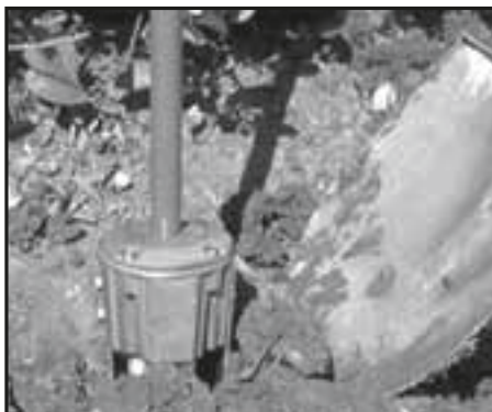
5. Fill hole with soil, concrete, or other permanent media to secure and support lighting fixture. Take into consideration the weight and height of the fixture and also the soil condition.
