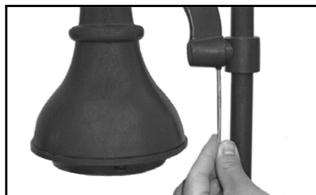
5. Loosen setscrew, adjust fixture rotation and tighten setscrew (300° rotatable).
