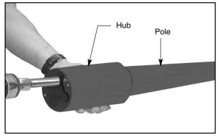
1. Install swept arm hub to pole with bolts, tighten to 20 ft.-lbs.
