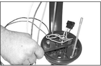
2. Install the fixturebase to down cast arm. Important! Keep wires tight when attaching fixture to arm to avoid pinching wires. See fixture installation instructions for fixture attachment.
