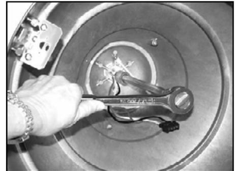
3. Install fixture head onto s-shaped up cast arm. **IMPORTANT! Keep wires tight when attaching fixture to swept cast arm to avoid pinching wires.**
