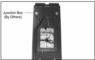
2. Securely mount wall plate over junction box (by others) on wall. CAUTION: Structural integrity of mounting plate attachment to wall is by others.
