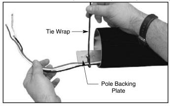
Lay pole horizontal on padded supports to protect finish. Pull wires through pole & out the top. Tiewrap wires to pole backing plate. Tie wires in a knot or back loop through tie-wrap. Wire leads need to extend 12" beyond the handhole.
