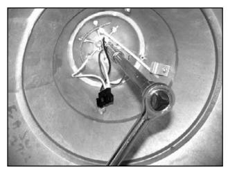
Install fixture head to side pole up swept cast arm with washers & nuts, tighten to 20 ft.-lbs.
