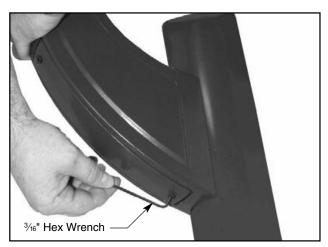
5. Push wires into pole and out pole handhole. Secure wire with the cable tie provided. Install arm access cover and secure with screws.
