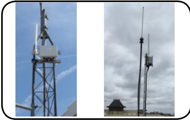
Example Roof Mount Structures
