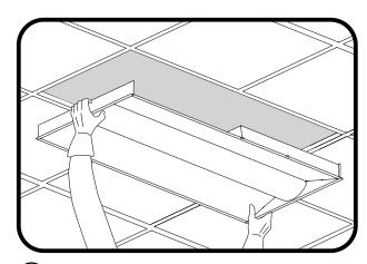
(2) Install the unit into the reserved hole in the ceiling.
