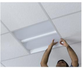
**STEP 2**To remove the lens squeeze one end of the lens until you can reach under the center and pull the lens out.
