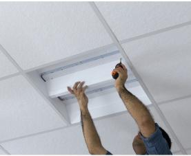
To reassemble reinstall the cover and replace the screws. Then install the lens by placing one edge into place and bending the other side to fit into place.
