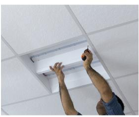
**STEP 3**To remove the cover remove the 4 screws and squeeze the cover to release.
