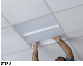
To reinstall lens, place one side of the lens against cover, squeeze lens and push up. Release lens and verify it is snug along housing.
