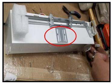
Place the bar hanger on the housing and align the bracket with the newly created holes
