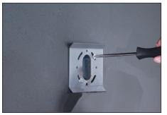
Remove the back mounting plate from the back of the fixture. Secure back plate to outlet box with provided 8-32 screws.
