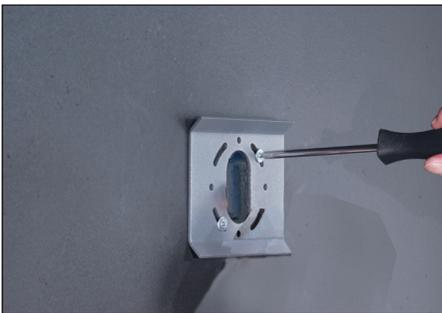
3) Remove the back mounting plate from the back of the fixture. Secure back plate to outlet box with provided 8-32 screws.
