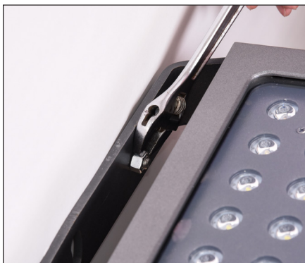
1. Secure fixture by tightening 1/2" bolts (2) place, torque nuts to 45 foot-pounds.
