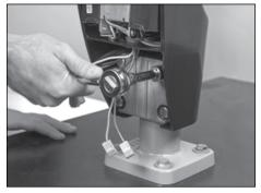
7. Add threadlocker fluid (i.e. Loctite\*) to (4) 3/8" hex bolts and tighten with 9/16" socket and ratchet. Casting has a ±5° tilt allowance for leveling. Tightening the top bolts first, angles the fixture towards rear. Tightening bottom bolts first, angles fixture forward. Tighten to 27.12Nm (20ft-lb).
