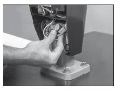
**8.** Make wire connections, black to voltage, white to neutral/common, green to ground. Bundle wires neatly above tenon clamp.
