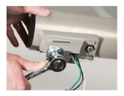
6. Tighten bolts on speed mount. Be sure speed mount is aligned with anchor base and other fixtures for multiple mounts. Tighten to 20 ft. lbs. using N" socket with ratchet.
