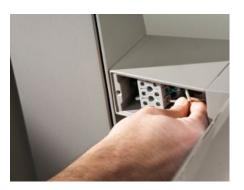
Connect wires (voltage to black, white to common, green to ground) directly into the terminal block.
