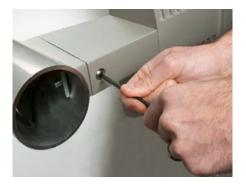
**8.** Tighten the top bolt in luminaire arm with J" hex wrench to secure luminaire to Speed Mount and pole.
