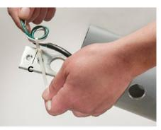
2. Lay pole horizontal on padded supports to protect finish. Pull field wires through pole and secure them with the tie-wrap (C) at the top of pole backing plate.
