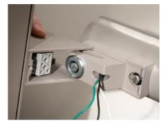
7. Attach the luminaire sliding the arm over the speed mount from the top of the pole.
