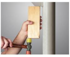
2. Place a wood block at base of luminaire arm and use a mallet to loosen fixture from Speed Mount.
