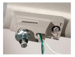
**5.** Thread top bolt through flat washer and shoulder washer, and bottom bolt through flat washer into pole backing plate inside pole.
