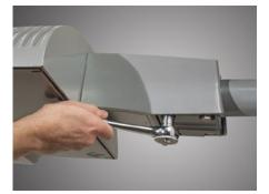
2. Add threadlocker fluid (i.e. Loctite\*) to (4) bolts and tighten bolts with N" socket and ratchet on the adjustable die-cast plate at bottom of slip-fitter arm to secure the luminaire.
