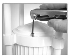
**14.** Install splice compartment cover with screws provided (2 places).
