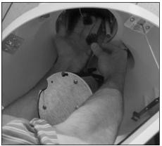
**2.** Connect incoming quick-disconnect to electronic driver and install driver tray through key-holes onto screws, tighten securely.
