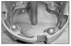
Install the base casting on the preset anchor bolts. Use flat washers and hex nuts both below and above the base casting.
