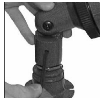
4. Loosen setscrew, adjust fixture rotation, and tighten setscrew. Connect fixture to main system cable with a KLV410 Sealed Connector. (See KLV410 Installation Instructions)
