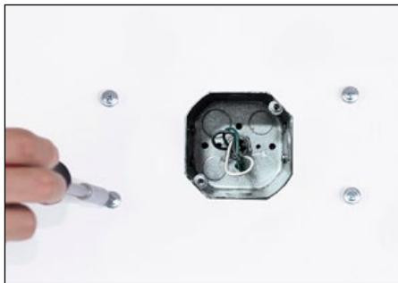
2. Install mounting hardware (do not tighten it).
