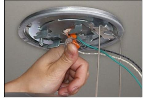
**5.** Push the electrical connections into the J-BOX.
