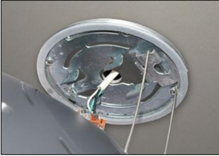
**3.** Hang the fixture on the speed mount bracket, allow fixture hang freely.
