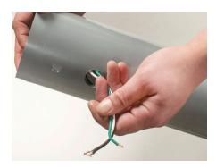
**3.** Push the pole backing plate into pole and run field wiring through the center hole in the pole backing plate. Wiring exits through the center of the three holes.
