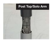
**4.** Use 9/16 socket with extension, expand the spreader to secure the fixture to the pole, torque to 20 lbs.
