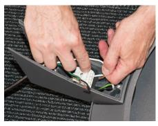
**10.** Connect wires (voltage to black, white to common, green to ground) directly into the terminal block.
