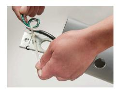
2. Lay pole horizontal on padded supports to protect finish. Pull field wires through pole and secure them with the tie-wrap (C) at the top of pole backing plate.
