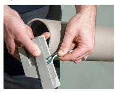
**4.** Pull wiring through speed mount. Make sure the wiring is long enough to reach terminal block on luminaire.
