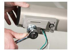
**6.** Tighten bolts on speed mount. Be sure speed mount is aligned with anchor base and other fixtures for multiple mounts. Tighten to 20 ft. lbs. using 9/16" socket with ratchet.
