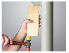
Place a wood block at base of luminaire arm and use a mallet to loosen fixture from Speed Mount.
