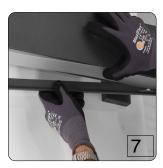
Put in lens latches. Repeat this step for continuous run.
