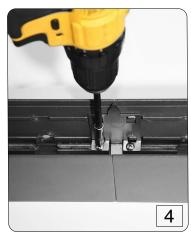
Align the next housing unit into the other half of the mating plate and repeating step 3.
