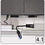
Continuous run: connect the mating power cable from one light engine to the other light engine. Repeat this process for multiple sections.
