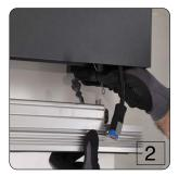
Attach retention cables to eyelets on both sides of the light engines.
