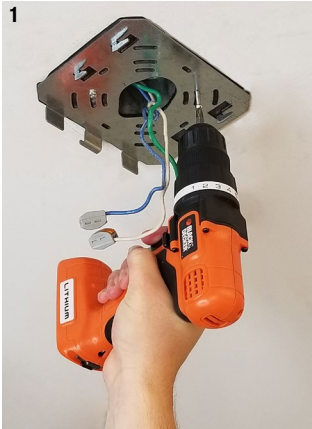
Mount plate to junction box.
